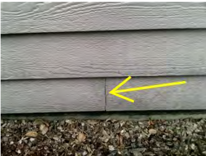
Photo 9-3 Deteriorated caulk at siding butt joint on south side.
