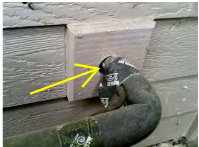
Photo 9-4 Deteriorated caulk at siding trim joint on south side.
