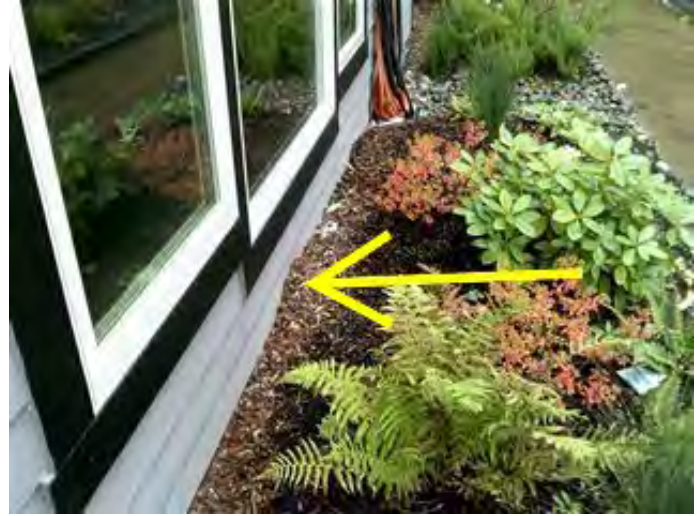
Photo 7-2 Earth siding contact on east side under master bedroom windows.
