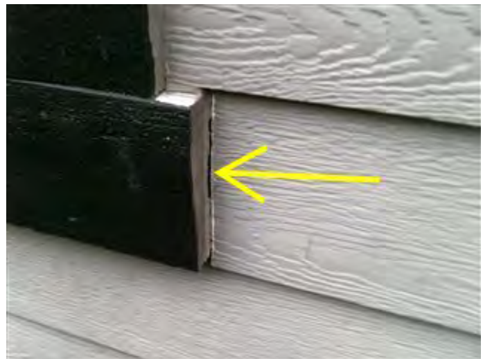
Photo 9-4 Deteriorated caulk at siding trim joint on south side.
