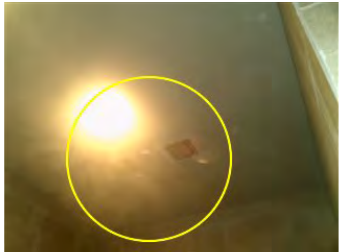
Photo 43-2 Water sprayed on ceiling when shower was turned on in shower #C.
