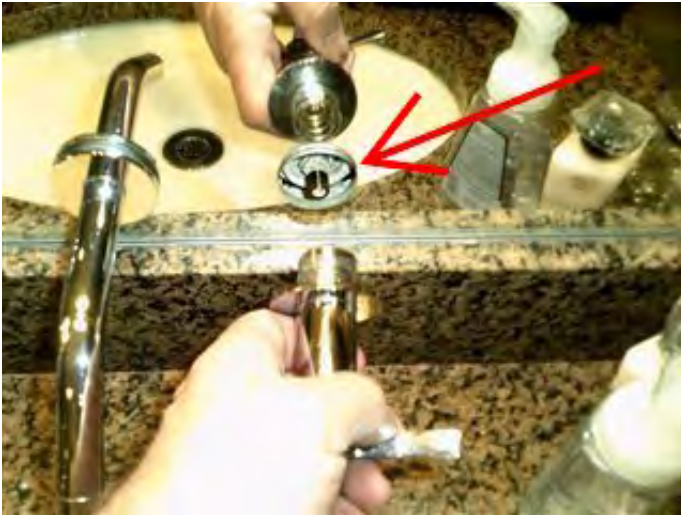
Photo 41-1 Master bathroom #C right sink.
