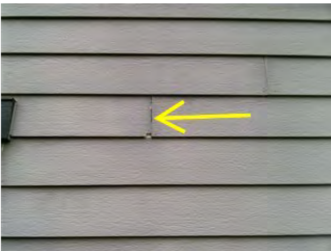
Photo 9-3 Deteriorated caulk at siding butt joint on south side.
