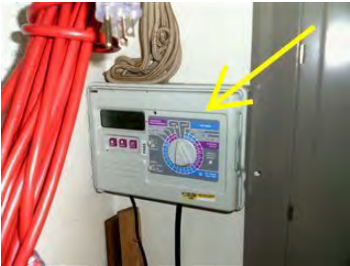
Photo 25-1 Sprinkler control.
