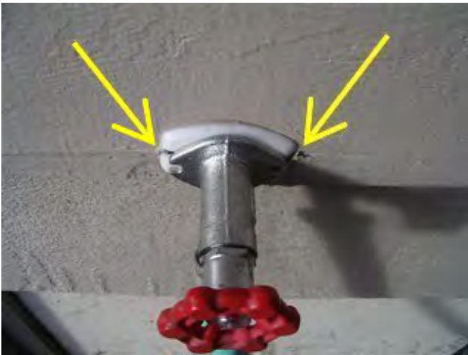
Photo 38-1 NW corner of garage.
