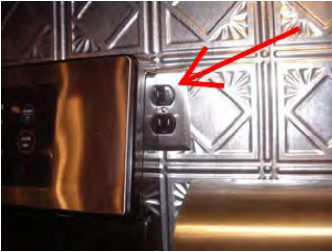
Photo 36-1 Receptacle partially covered by range.
