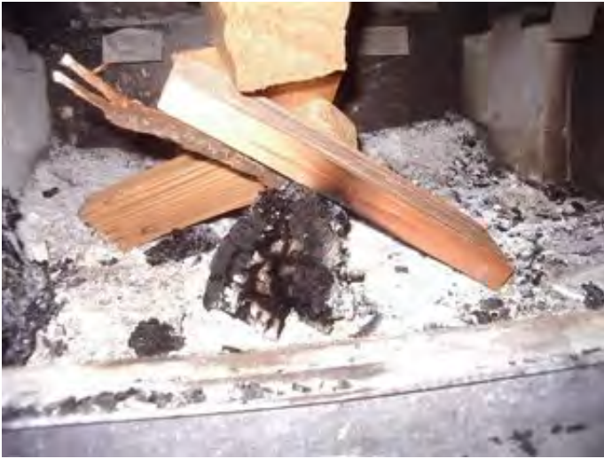
Photo 55-1 Fire materials blocking view.
