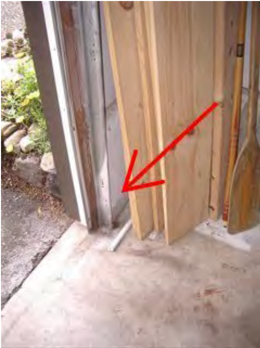
Photo 25-1 No photoelectric sensors.
