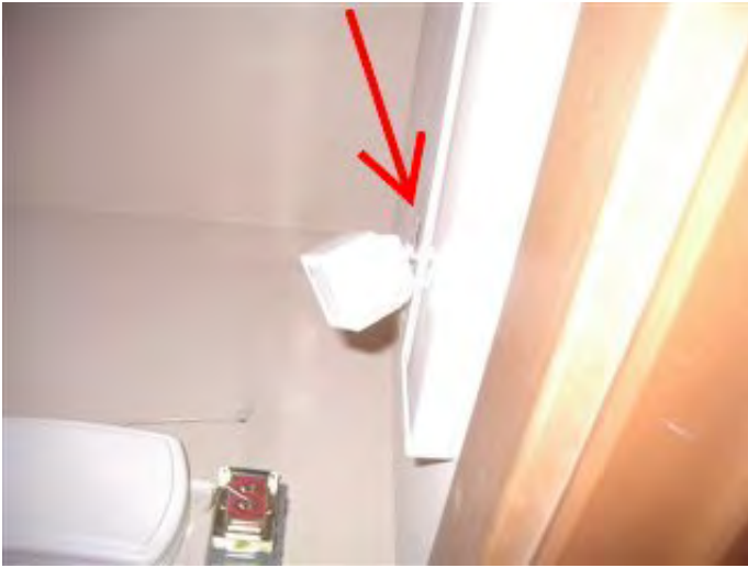
Photo 6-1 Loose motion sensor on light in entry coat closet.
