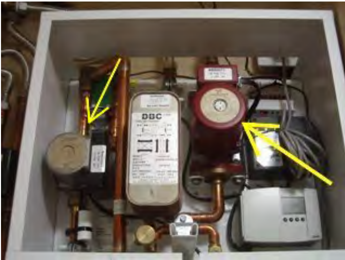
Photo 10-1 Circulating pumps.
