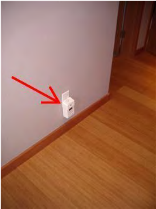
Photo 4-1 Plug in CO alarm.
